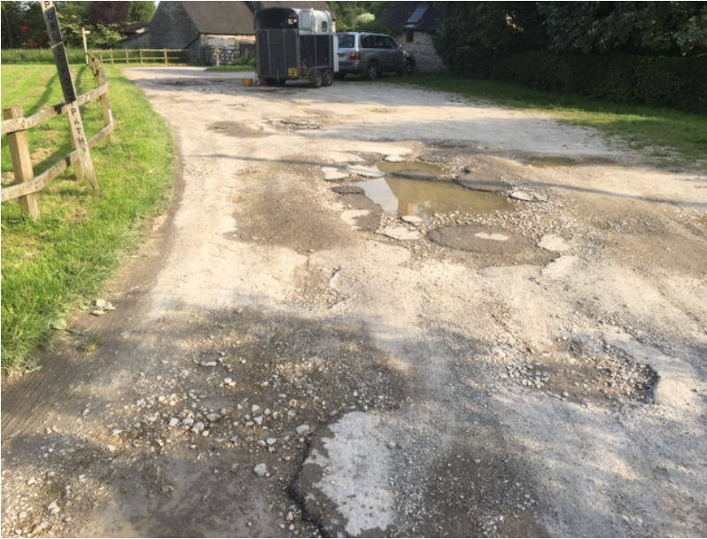
View from entrance showing Blanch Meadows in the background June 2017
