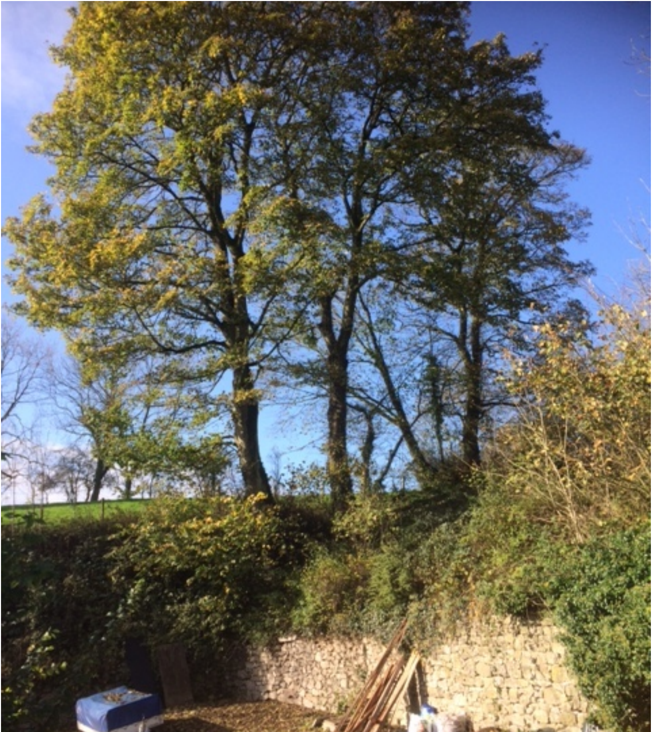
Trees above retaining wall at Millennium Green (note 2)
